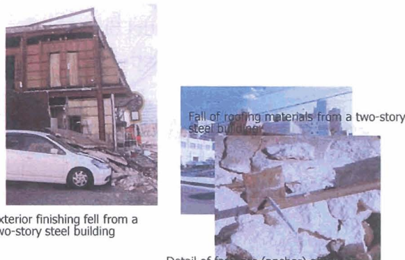
Detail of fastener (anchor) of failed ALC exterior wall
